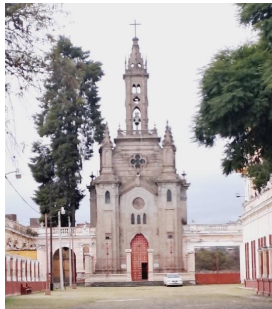
Figure 1 Façade of the El Carmen Church
