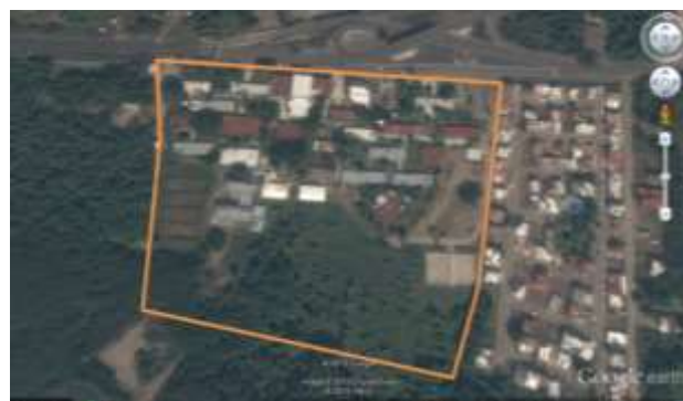
Figure 1 Campus Manzanillo, 400 kWp
