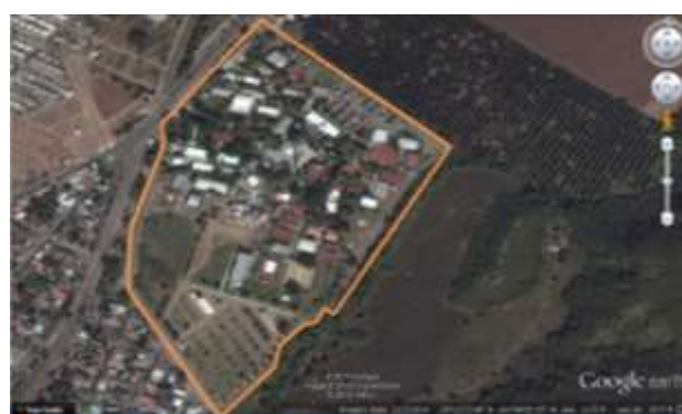
Figure 4 Campus Coquimatlán, 500 kWp
