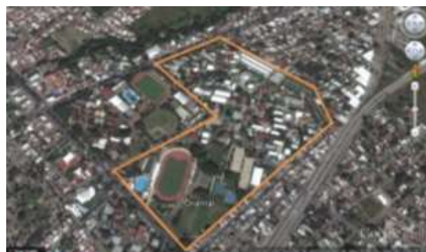
Figure 3 Campus Colima, 800 kWp
