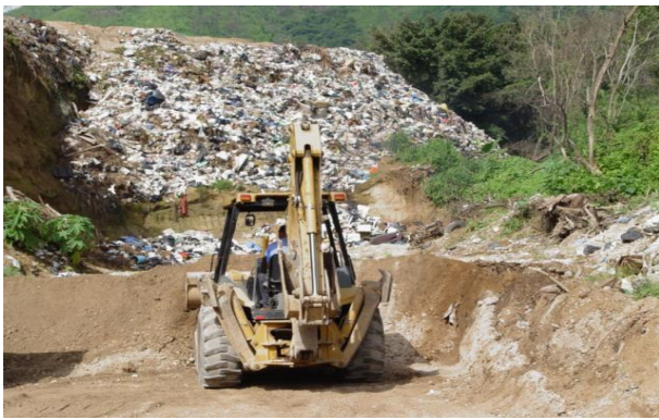
Figure 2 Natural soil where solid waste is deposited, showing the lack of the geomembrane (Murray 1999)
