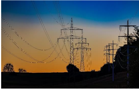
Figure 2 Overhead transmission lines
