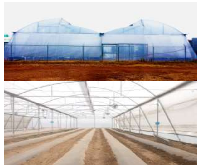
Figure 1 Indoor and outdoor view test greenhouse
